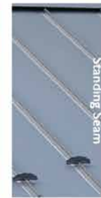
Metal Roof with Snow Guards
